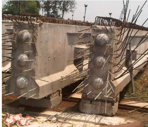
b) Cementitious end-caps used in a girder
