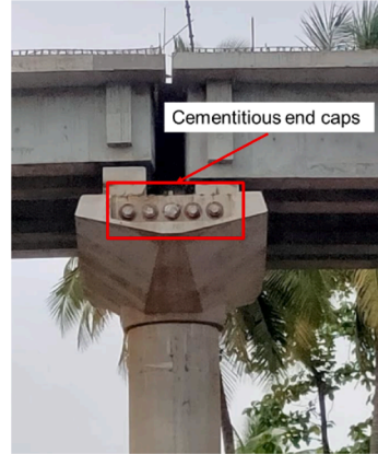
c) Cementitious end-caps used in a metro bridge
